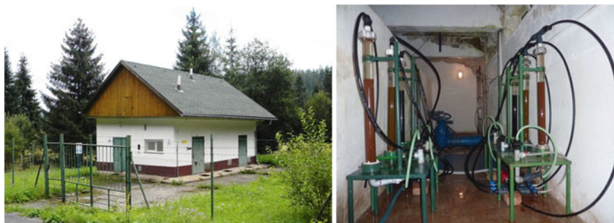
Fig. 5 Dúbrava chlorination plant and model filtration columns
